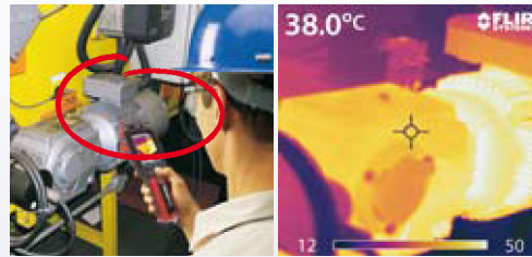
Mechanical check-up of an electrical motor using the FLIR i60.
